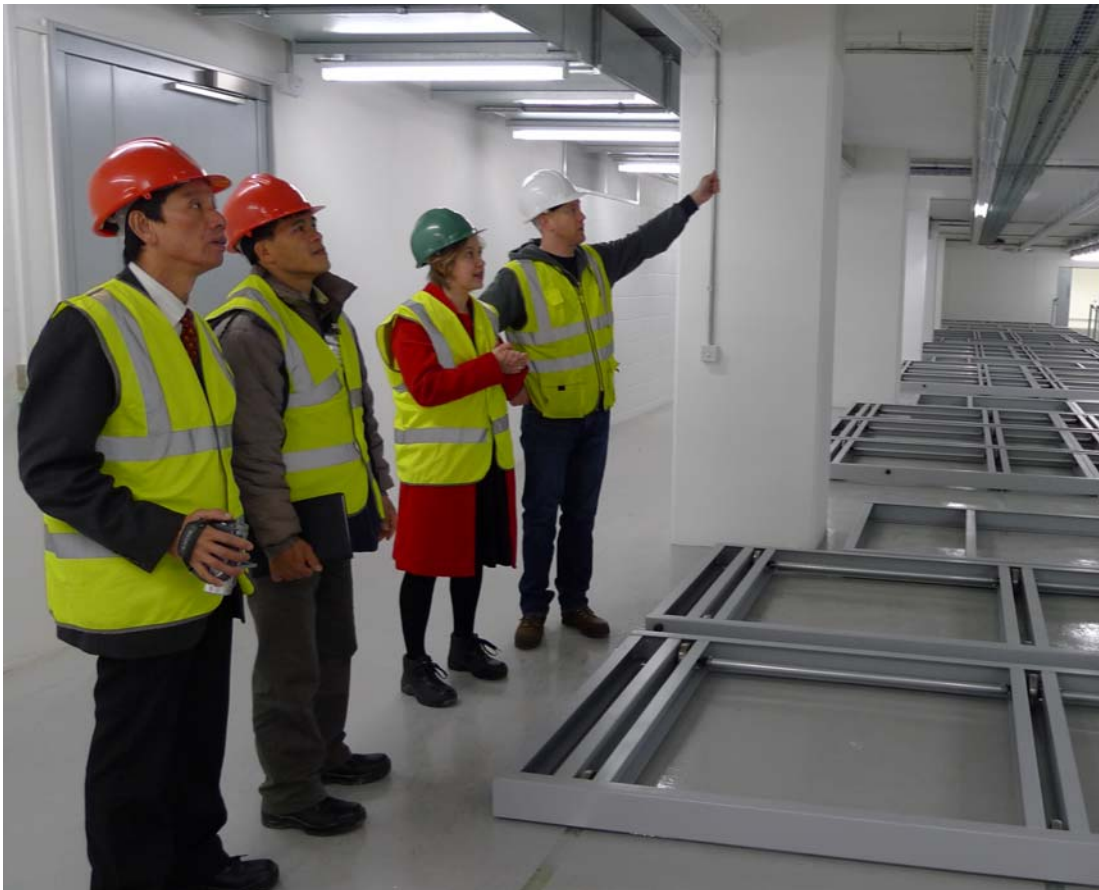
Figure 32. Viewing the collections' storage area under construction at the NHM Darwin Centre.
